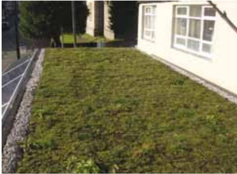
Lindum's green roof package consists of vegetation layer, plus GT4 substrate, which contains award-winning recycled topsoil, and Roofdrain drainage layer (incorporating a geotextile filter membrane), to sit above the waterproof membrane.
